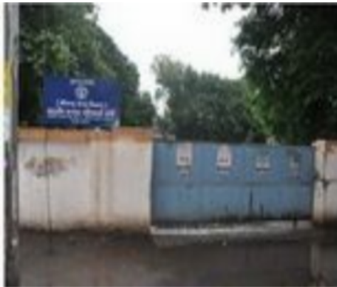
Polling Station Building Front View
