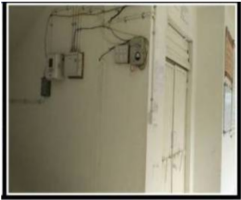
Polling Station Front View
