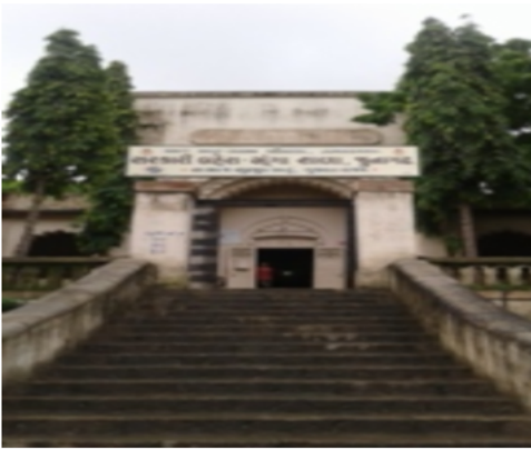
Polling Station Building Front View
