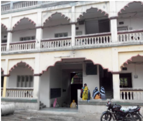
Polling Station Building Front View
