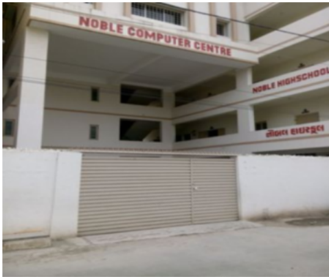
Polling Station Building Front View
