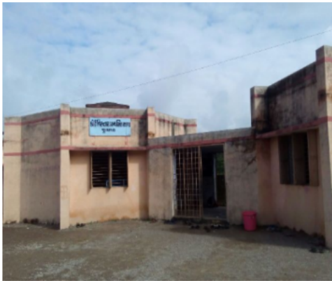
Polling Station Building Front View
