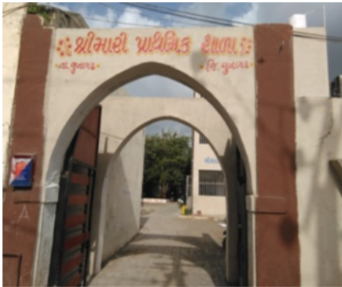
Polling Station Building Front View
