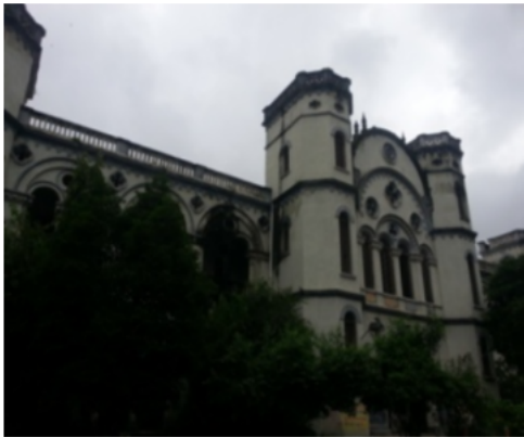
Polling Station Building Front View
