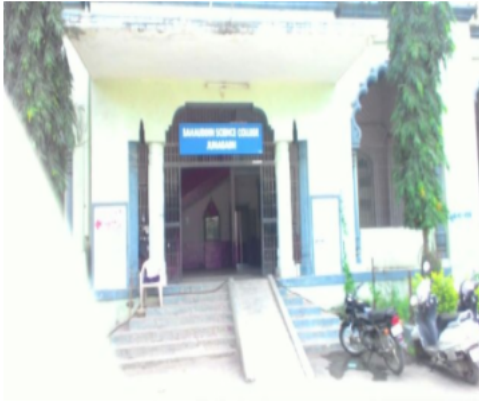
Polling Station Building Front View
