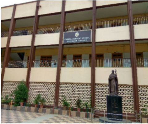
Polling Station Building Front View
