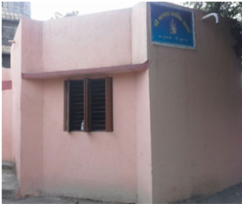
Polling Station Building Front View
