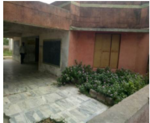
Polling Station Front View
