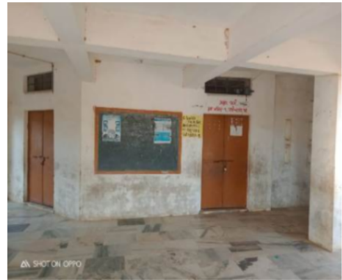
Polling Station Front View
