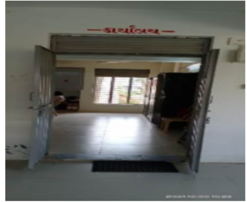
Polling Station Front View
