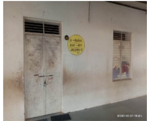
Polling Station Front View
