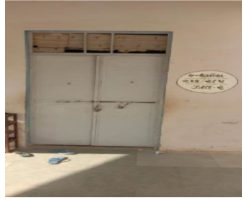
Polling Station Front View
