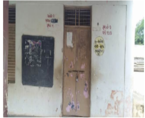
Polling Station Front View
