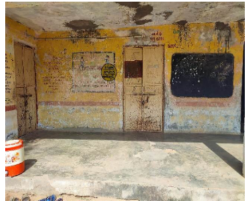
Polling Station Front View
