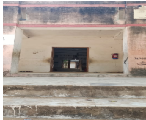
Polling Station Front View
