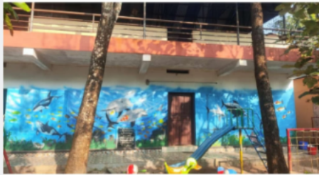
5* TOWN UPS KEERIKKAD NORTH BUILDING SOUTH WING
