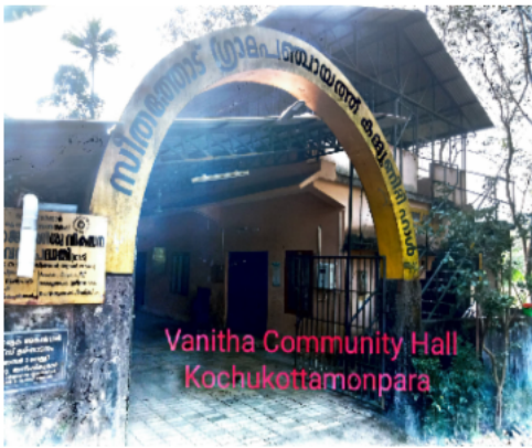
Polling Station Building Front View
