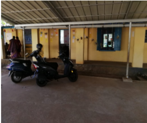
Polling Station Building Front View
