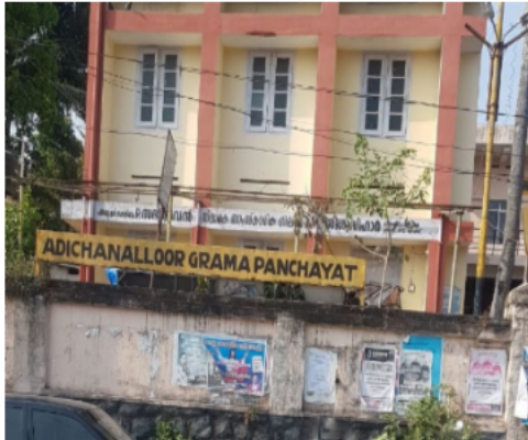
Polling Station Building Front View
