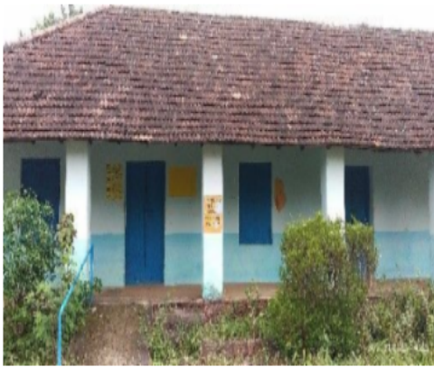
Polling Station Building Front View
