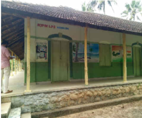
Polling Station Building Front View
