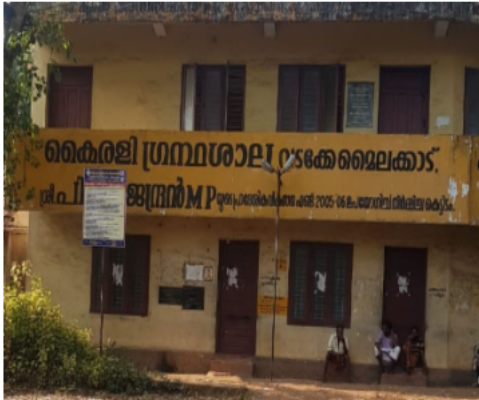
Polling Station Building Front View
