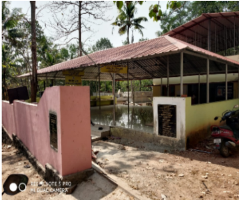
Polling Station Building Front View
