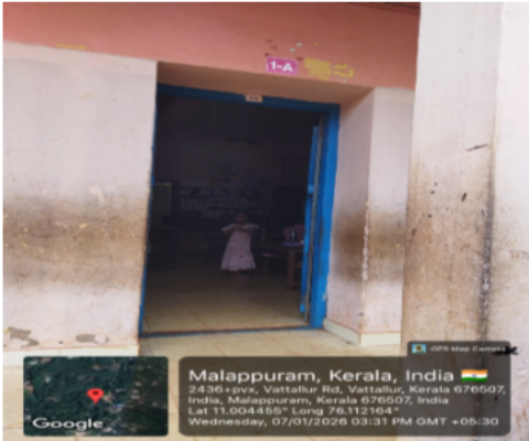
Polling Station Front View
