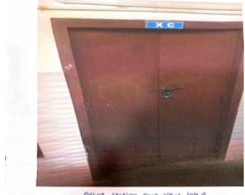
Polling Station Front View 104 A
