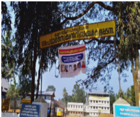
Polling Station Building Front View
