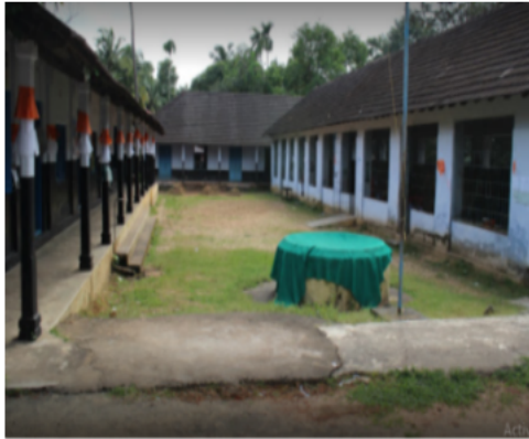
Polling Station Building Front View
