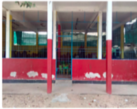
Polling Station Building Front View
