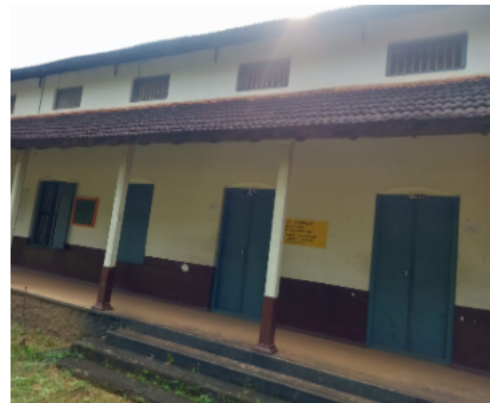
Polling Station Front View
