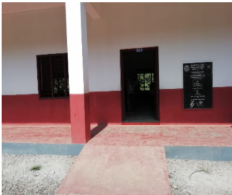
Polling Station Building Front View
