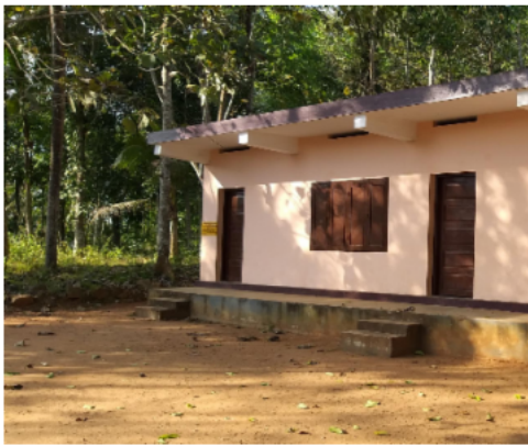
Polling Station Building Front View
