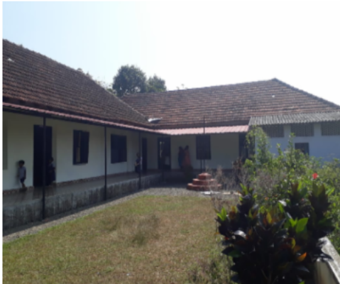
Polling Station Building Front View
