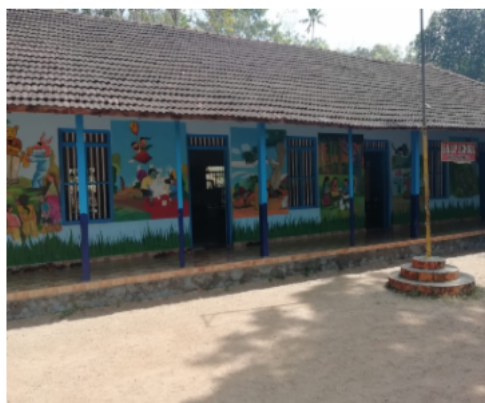
Polling Station Building Front View
