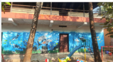
5* TOWN UPS KEERIKKAD NORTH BUILDING SOUTH WING
