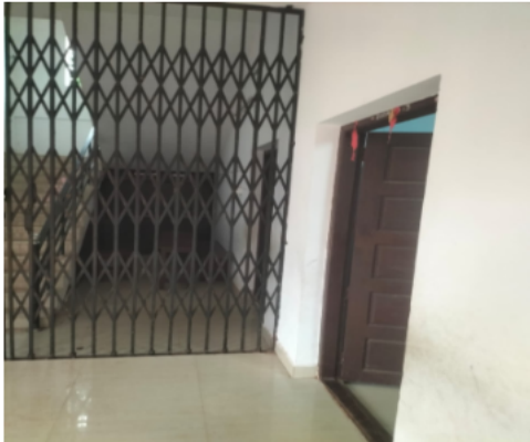
Polling Station Building Front View
