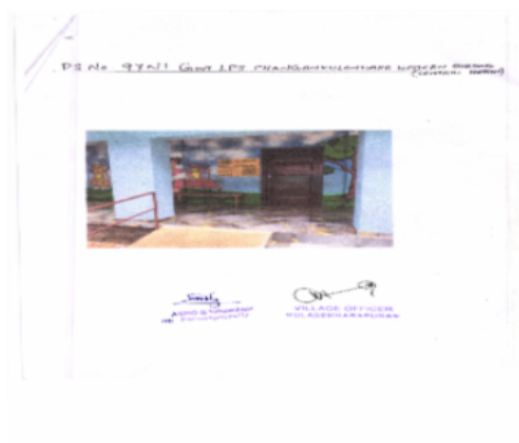
Polling Station Building Front View
