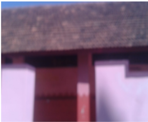
Polling Station Building Front View
