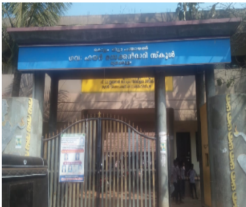
Polling Station Building Front View
