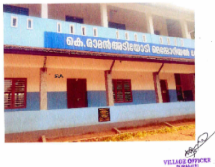
PS No: 58A (Proposed) Aroor UP School New Building East side.
