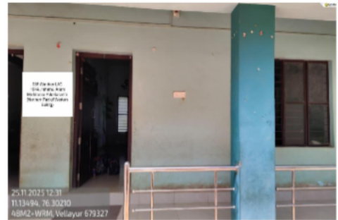
036 Wandoor LAC 154A Jirathathil Anam Madrassa Palakkalvetta (Northern Part of Western Buidlg)
