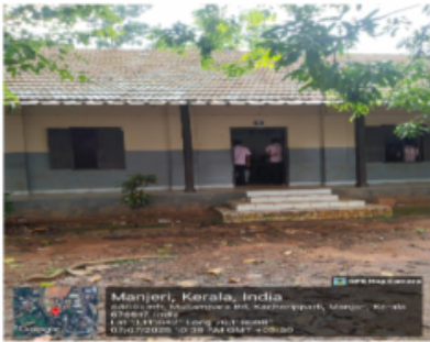
Proposed new Polling Station - 107A ( Govt. Boys Higher Secondary School, Manjeri - Corner of Old Building)
