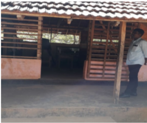
Polling Station Building Front View
