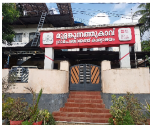
Polling Station Building Front View
