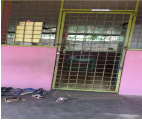
Polling Station Building Front View
