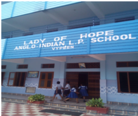
Polling Station Building Front View
