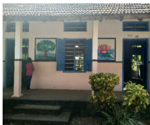
Polling Station Building Front View
